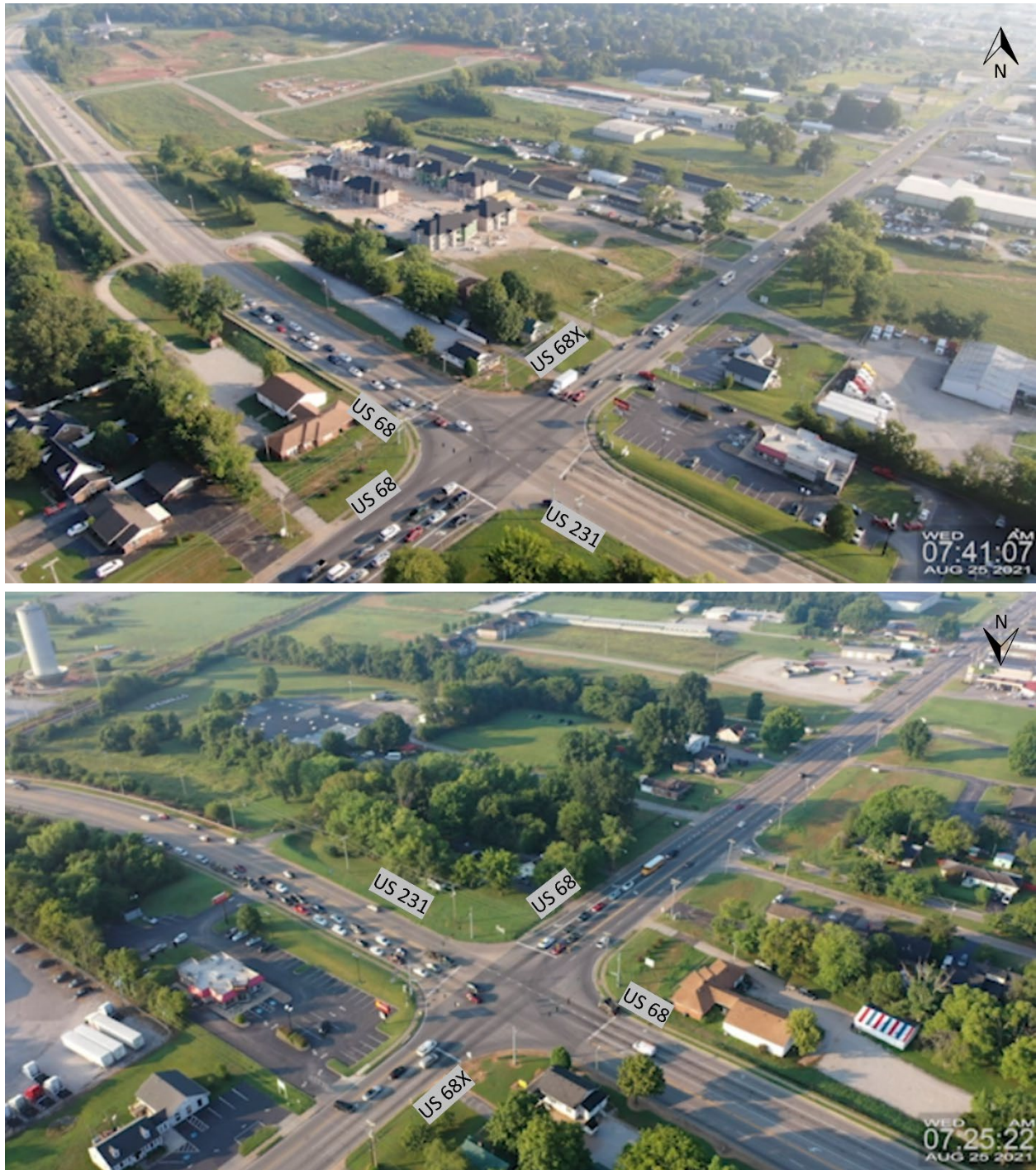
Figure 3: Drone Observed Maximum AM Queue Length
